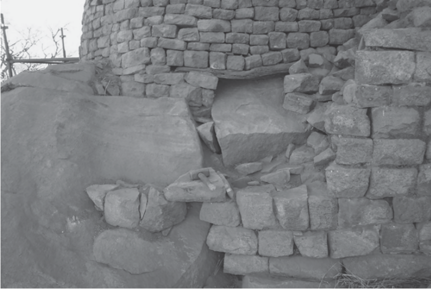
Figure 5.4 Wood used as a lintel over an irregular boulder, Cross Ruin, Khami Source: A. Sinamai
